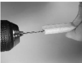
7. Drill two holes in top of strut.
